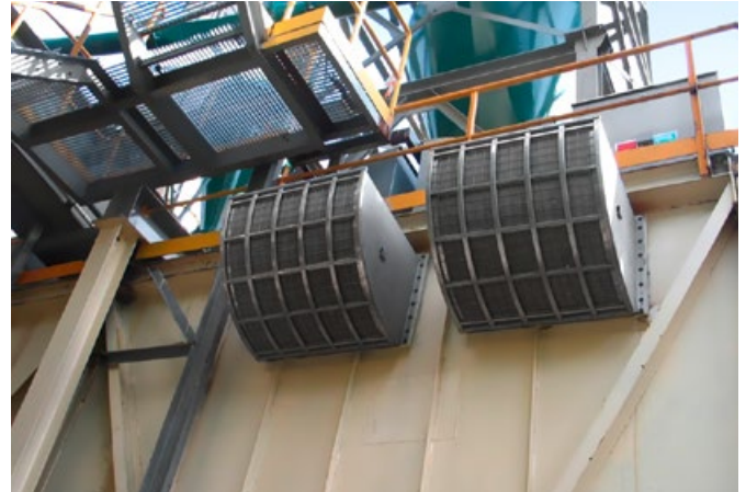
Explosion venting of a chip bunker using the Q-Box to protect the surrounding infrastructure.
